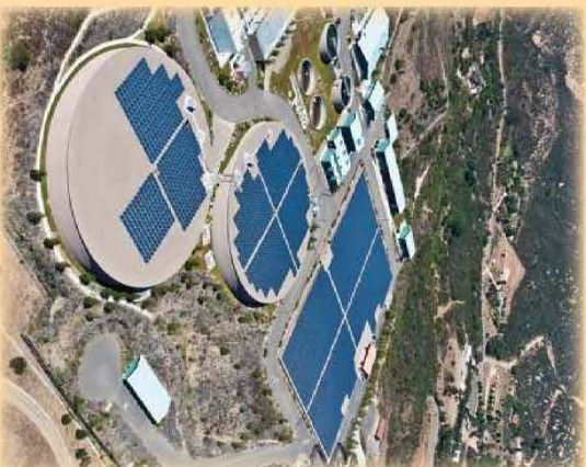
Twin Oaks Valley Water Treatment Plant $179 million
