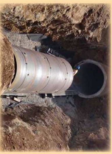
Pipeline Relining $786 million
