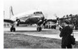
| 1949 Parallel runway system completed.
